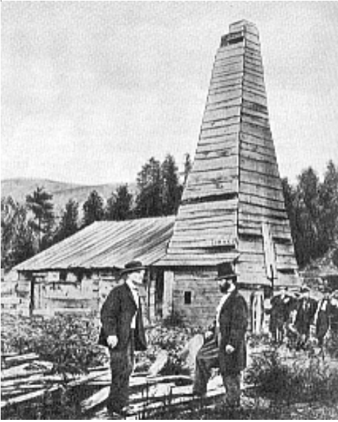
Fig. 1 — As Civil War started, first well drilled to obtain oil.
